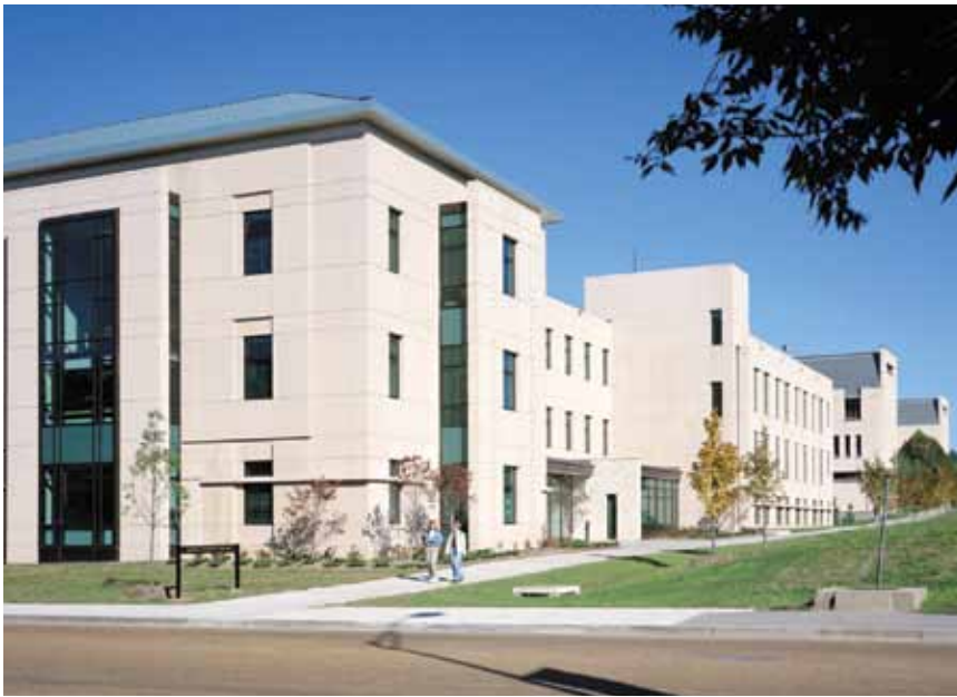
The four-story, 100,000 sq. ft. Anheuser-Busch Natural Resources Building's precast concrete façade houses offices, laboratories, and a 500 seat auditorium at the University of Missouri – Columbia.
